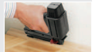
Using the ME 30/08 for invisibly countersinking brads when fixing skirting boards
